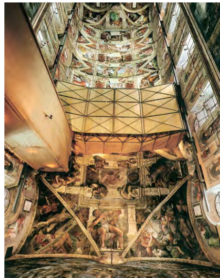
Restoration project with scaffolding
